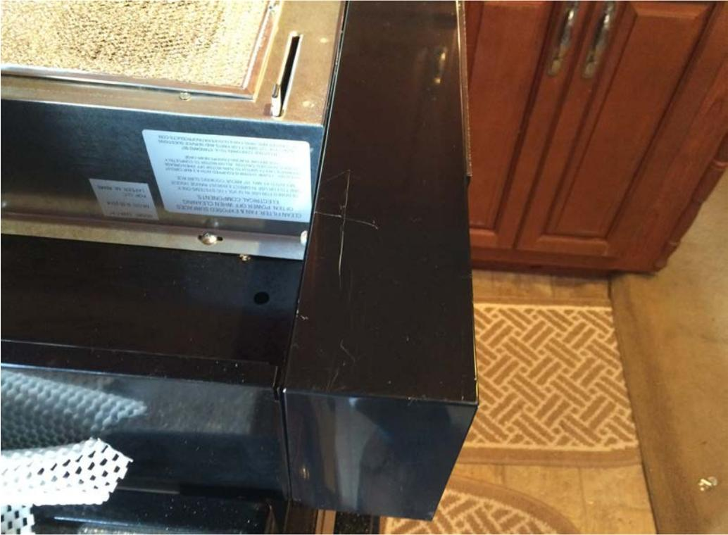
I set the hood on a box to facilitate the connections of the wiring. I also used the piece of wood support the back of the hood while I inserted the mounting screws. The brighter light is actually usable for cooking and the fan is much quieter. A great improvement to our rig!
