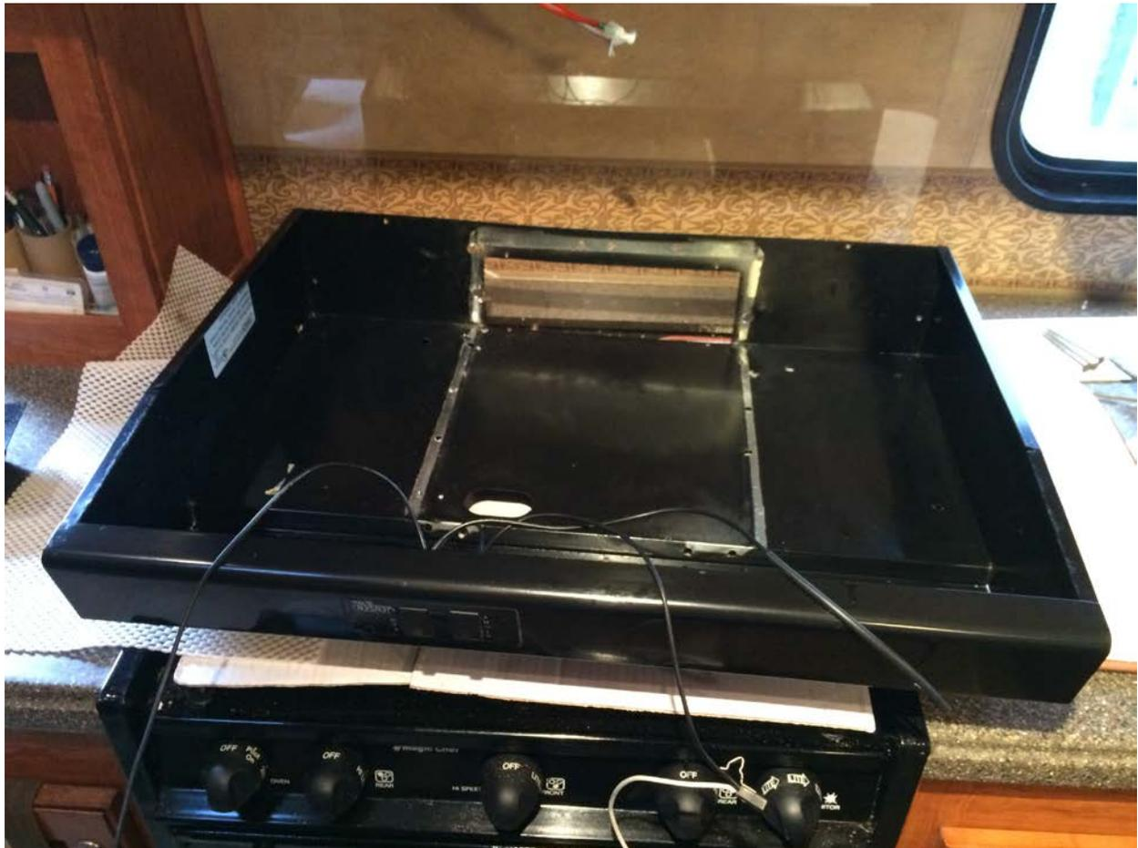
The fan box installation was simple and quick. The black wire from my hood switches connected to the plug as described on the instructions. I had to double check which wire came from the fan switch and light switch since the hood was upside down at this time.
